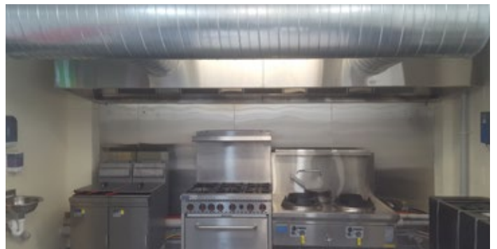
CNSST Community Kitchen Built by 30 May 2017
